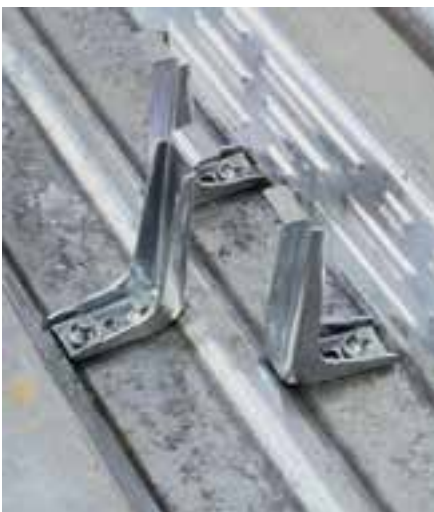
Figure 6: Hilti X-HVB installed on profiled deck
