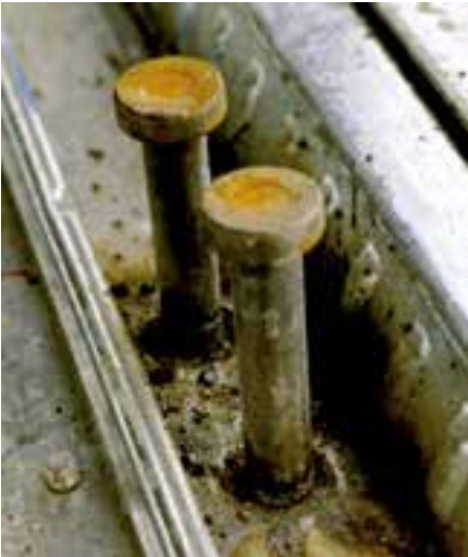
Figure 5: X-HVB shear connector in rehabilitation
