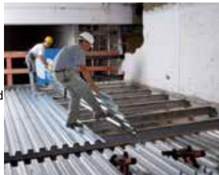
Figure 26: Installation phases for X-HVBs on profiled sheeting (from top left clockwise):
