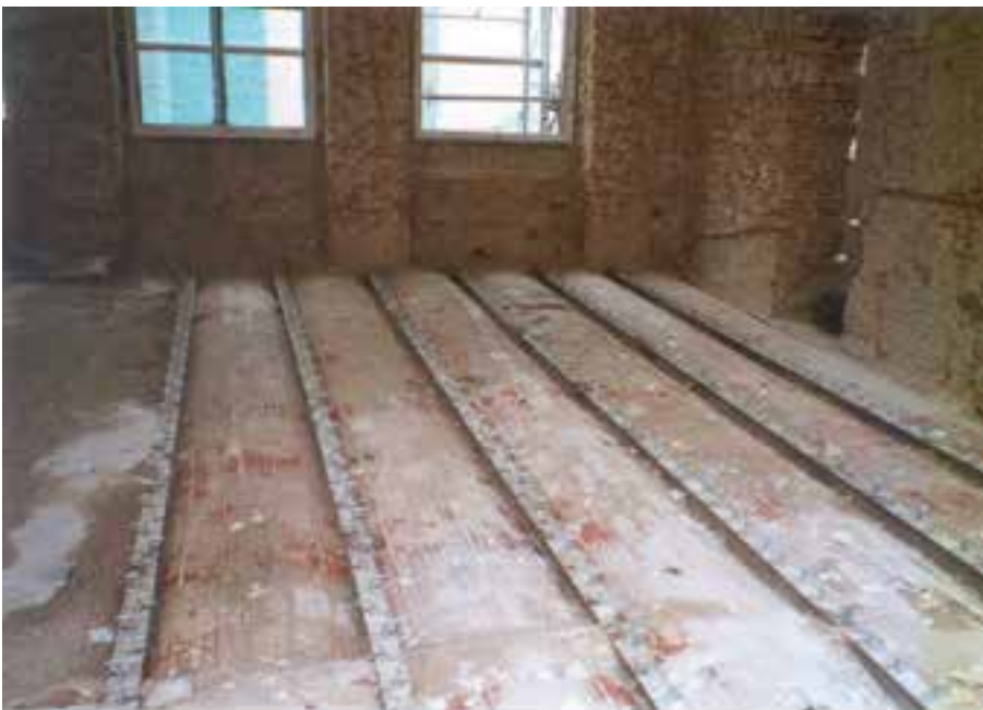
Figure 27: Existing slab to be strengthened by an additional thin concrete layer
